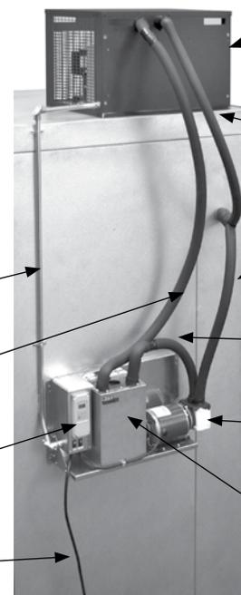
Photo shows BLC-1/3 in an installation setting with the control panel installed remotely from the condensing unit cabinet.
